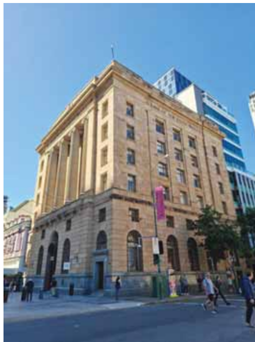
Figure 2 - The location of SOA's former office in the Bank of New South Wales Building. It is at the western end of the Queen St Mall.
