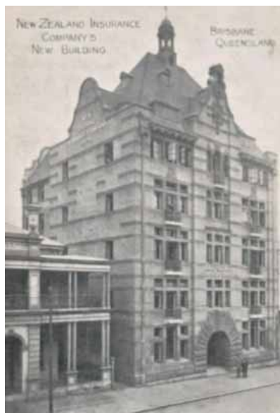
Figure 12 - A1909 photo of 334 Queen St 9 . The building would have looked essentially similar to this during the war.
