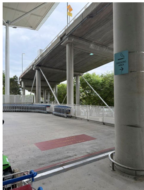
Level 2 Southern Slab – Trolley Drop Off Zone
